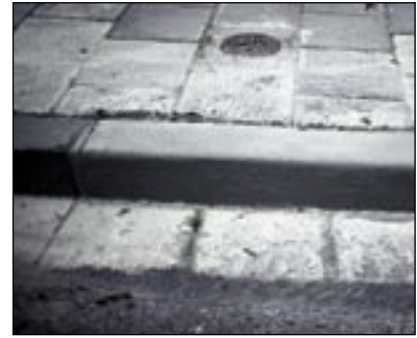
Repairing the kerbs with SILIKAL® Mortar R 17
