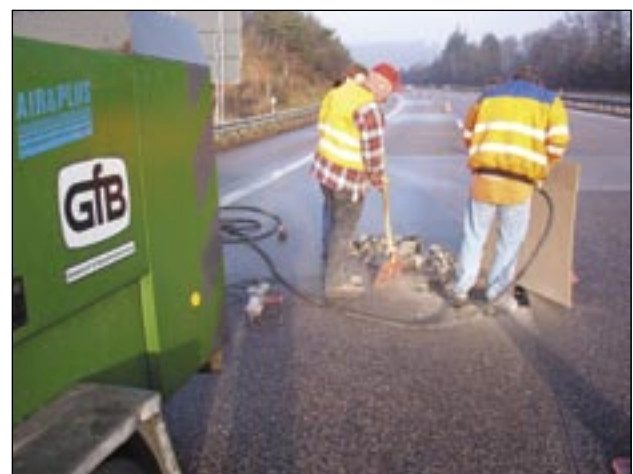
A3 Motorway, Neustadt/Wied: Improving the road surface
