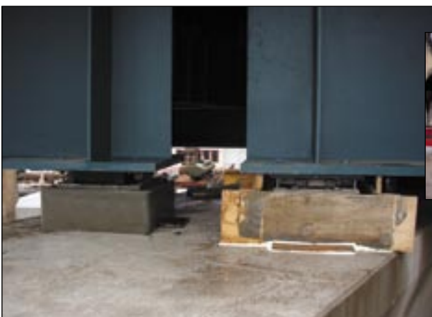
Chemnitz-Einsiedel viaduct, Blankenauer street: repairing bridge bearings
