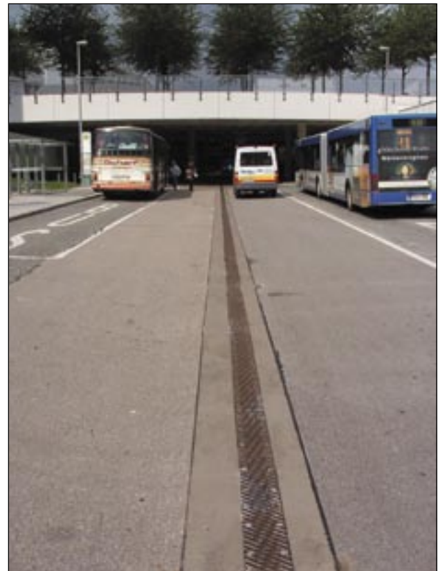
South bus station of the "Franz-Josef Strauss" airport, Munich: Repairing drainage channels
