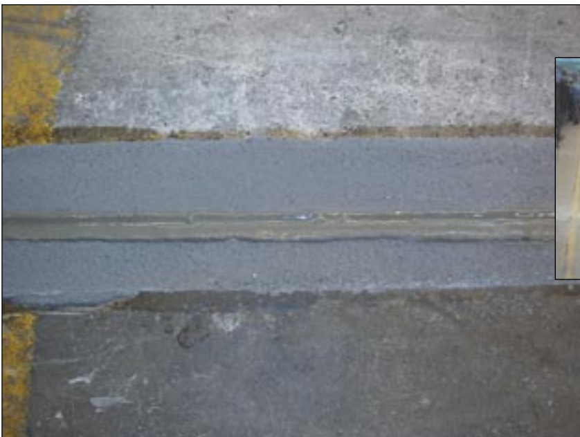
Left: Rheingas AG, Brühl: Repairing sliding gate
