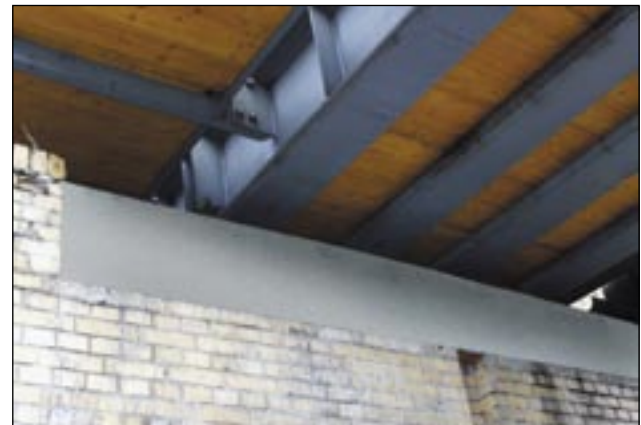
Metropolitan viaduct, Berlin, Sterndamm: repairing bridge bearings
